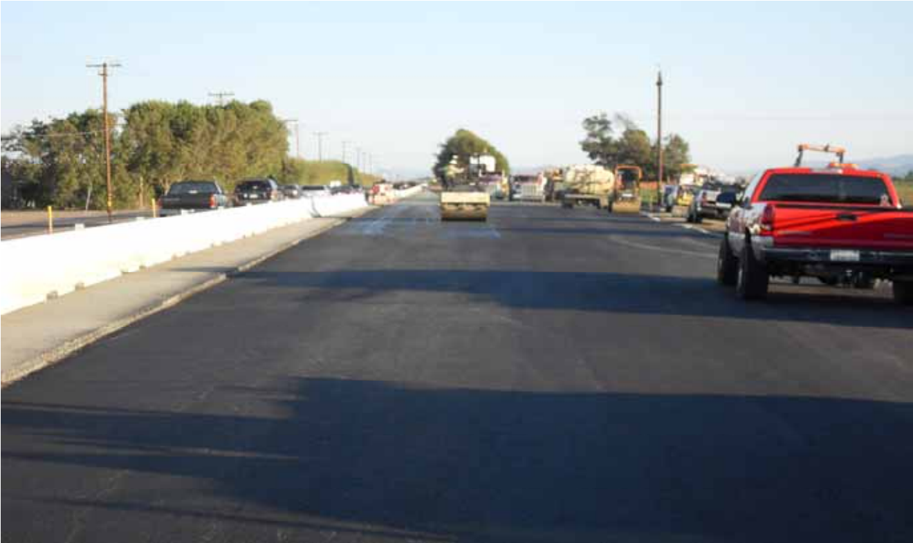
Pavex Paving at Hudner Ln.
