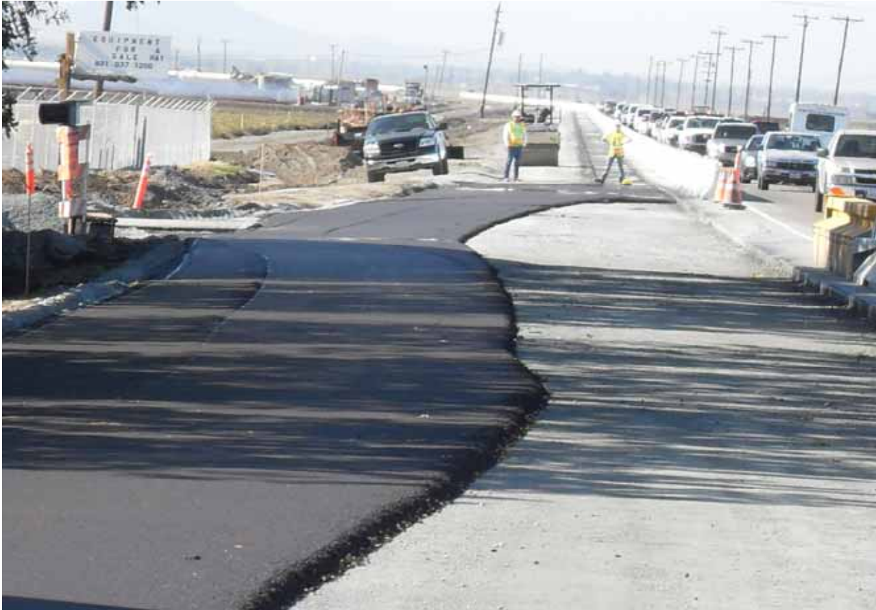
Pavex Paving Widening at Hudner Ln and compaction testing being performed.
