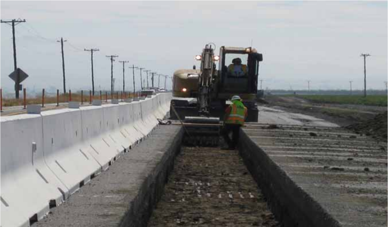
Pavex Digging Traveled Way Section
