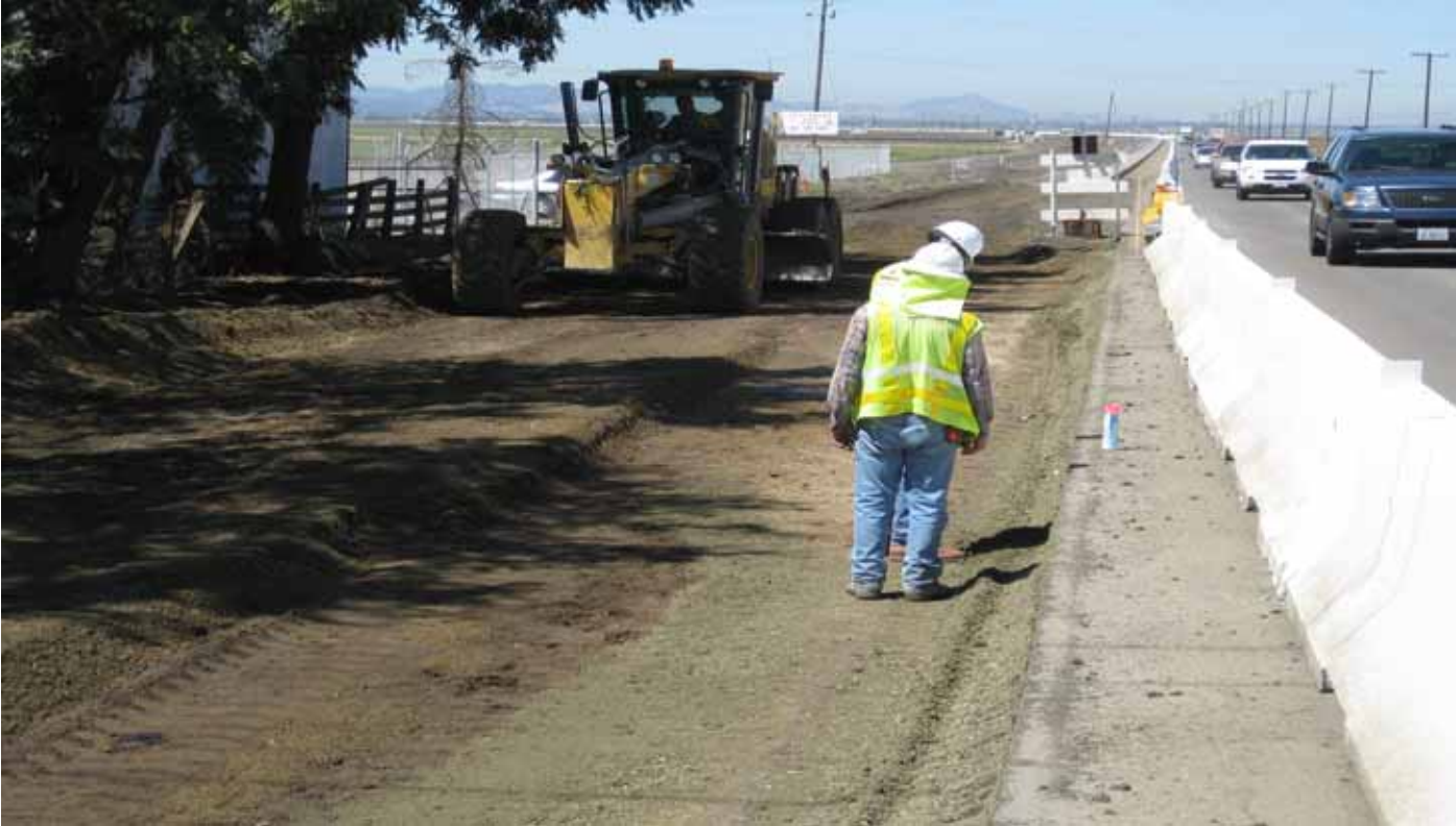
Pavex Grading at Hudner Ln.
