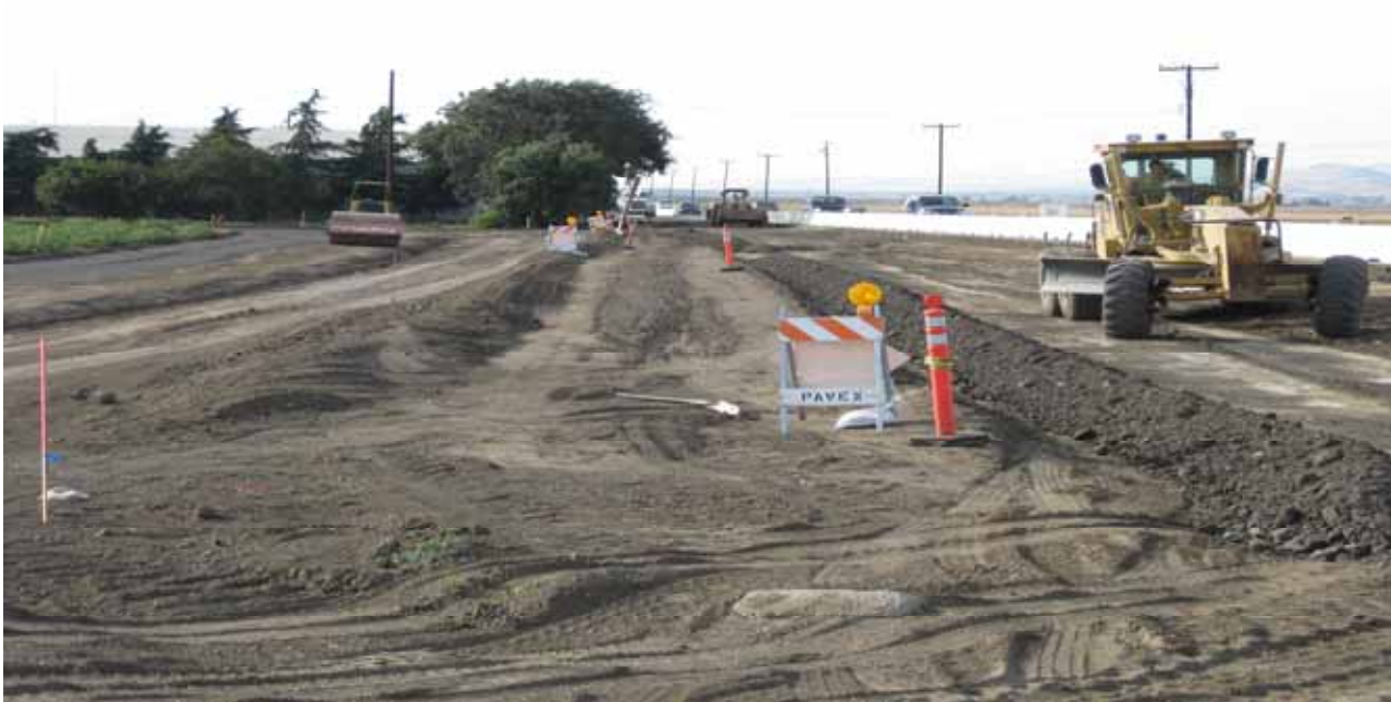
Pavex Grading Widening Intersection and Turn Lane at Hudner Ln.
