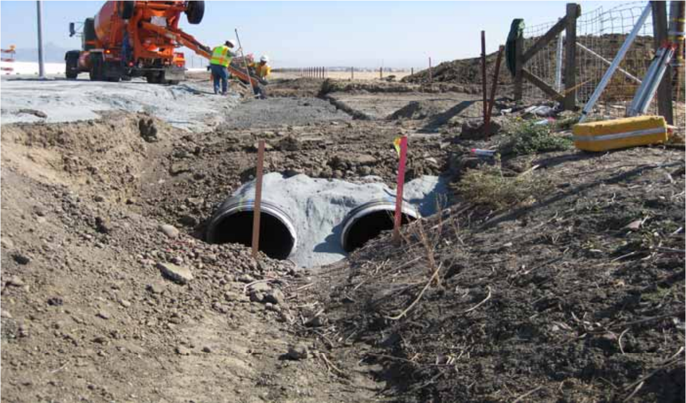
Pavex Installing Drainage System
